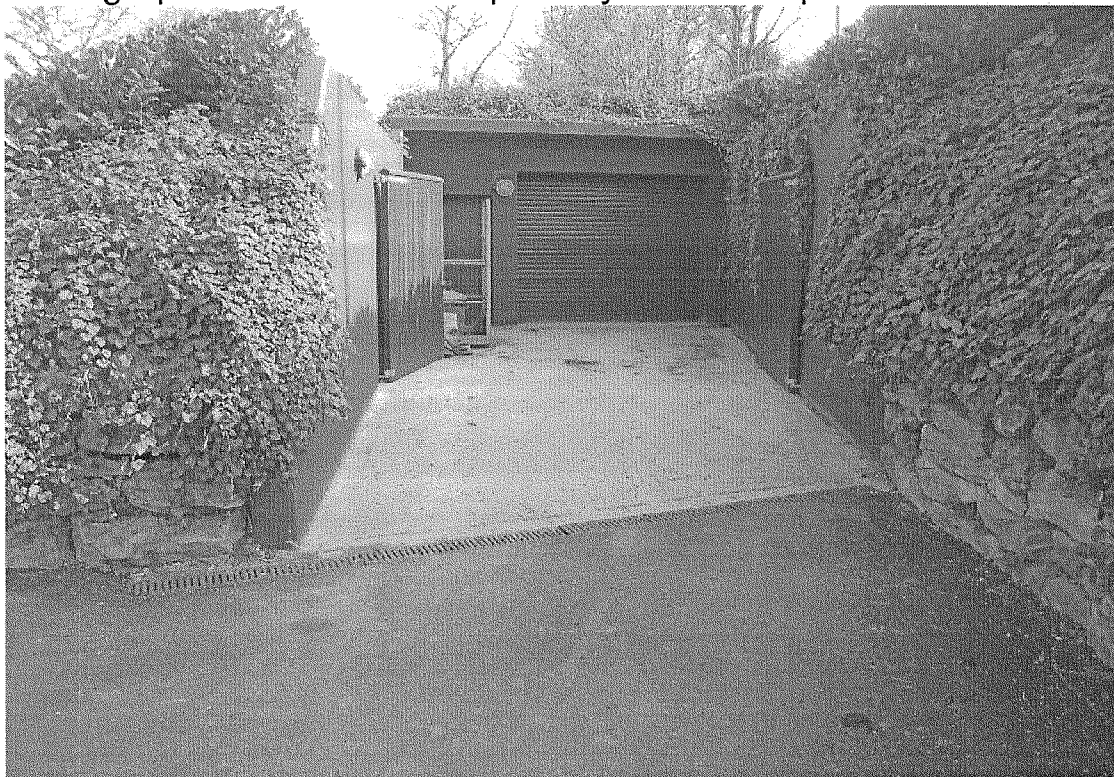
Photograph TP3. Erection of partially sunken implement store.
